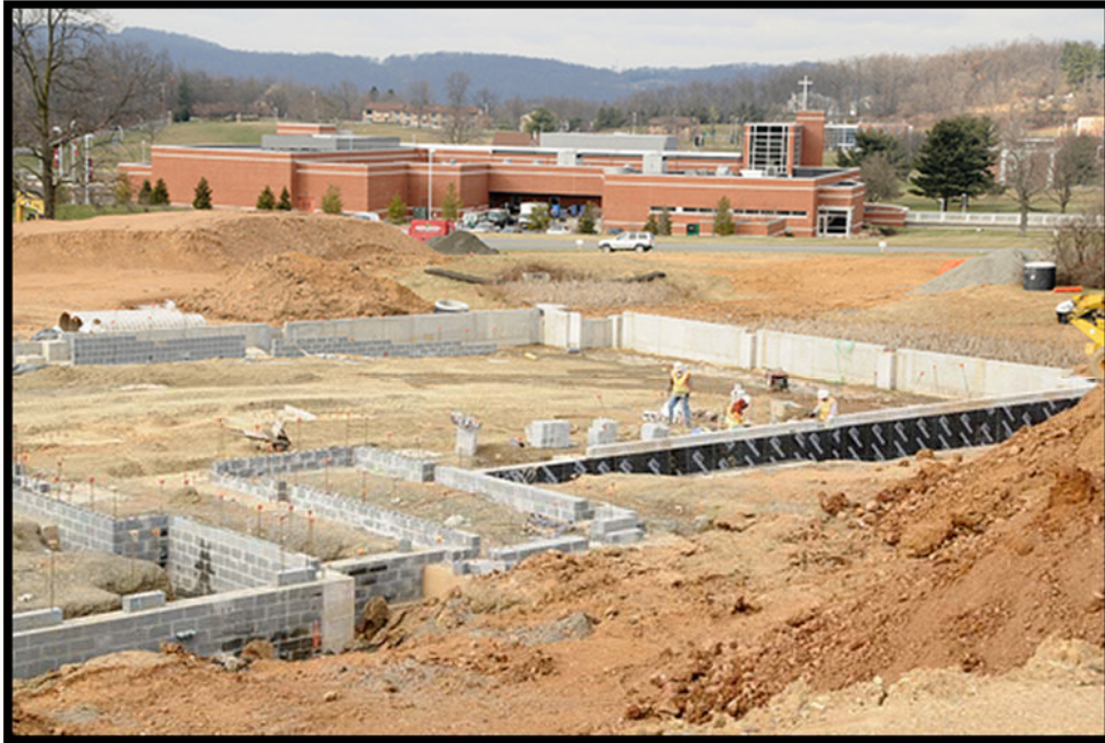
Figure 1: Footing Excavation and Constructed Foundation Walls
