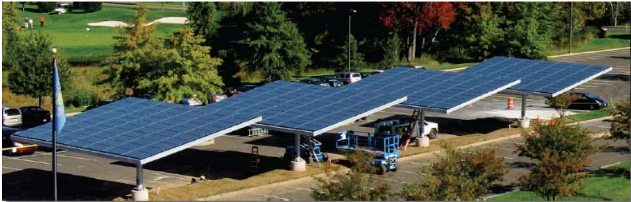
Figure 24: Envision Solar Tree® Parking Lot Solar Arrays
